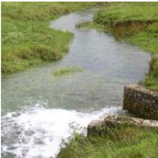
Stream support system pumps groundwater into a river to increase the flow
